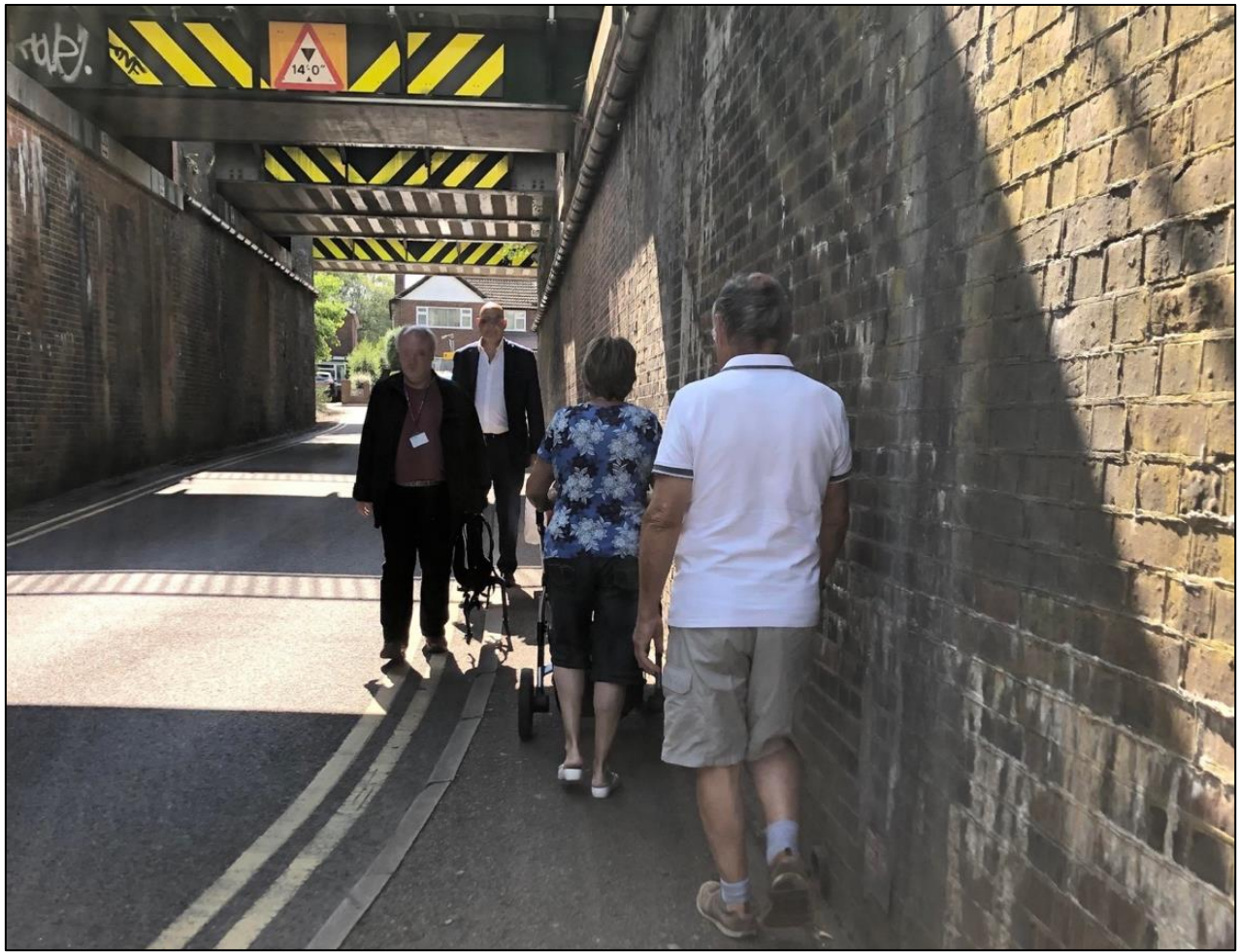
Figure 62 Pedestrian congestion under railway bridge
