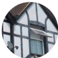
HALF-TIMBERED UPPER FLOOR
