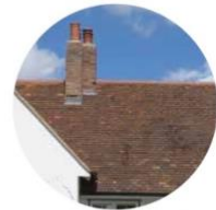
CLAY ROOF SHINGLES
